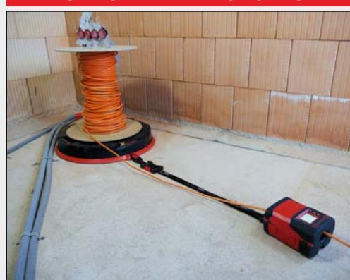
RUNPOMETER RM35 with **belt and clip system** connected to XB 500
