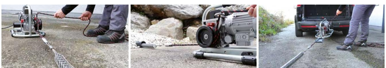
The operator stands next to the capstan winch with a sufficient safety distance and pulls with little effort at a 90° angle to the pulling direction on the pull rope. The effort should only be so strong until the feed rate is reached. **Very strong pulling does not increase the pulling power of the capstan winch!**
